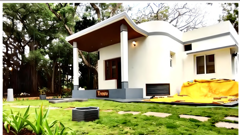
A 3D printed house at IIT-Madras, Chennai, Tamil Nadu, India (Source: TVASTA)
